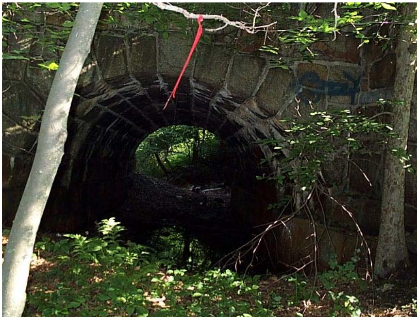
Photo 1: Looking north at the existing P&W arch. Photo date: July 16, 2006
